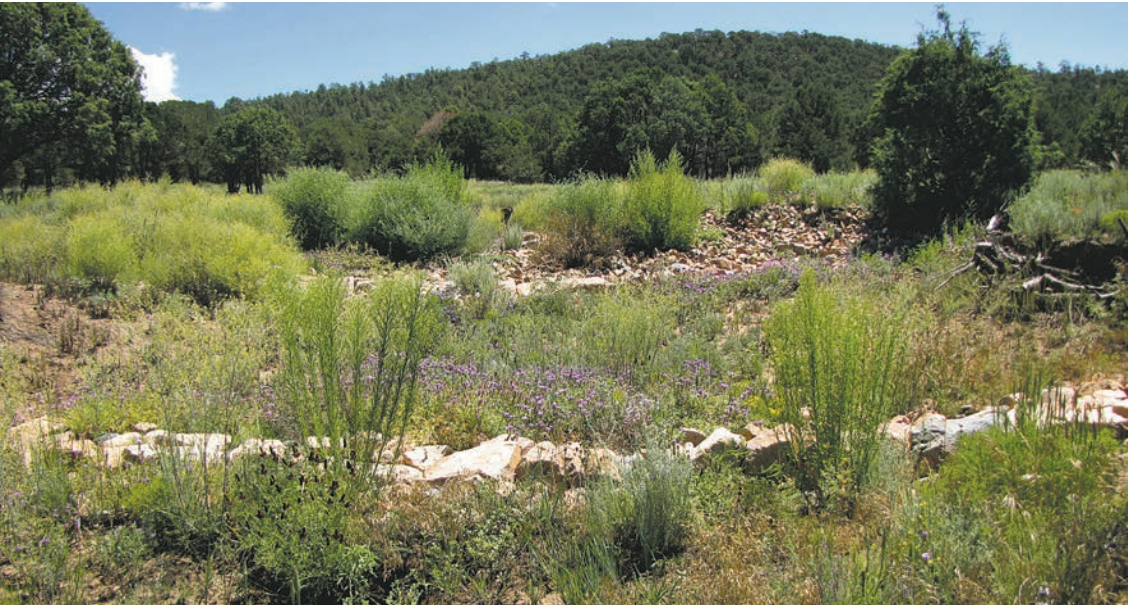
Examples of large One-Rock-Dams (foreground) and a Filter dam (background) in a stabilized rehabilitated arroyo and restored forest meadow.
