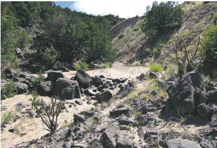
Example of rock dam holding back sediment in a steep arroyo (the arroyo crosses an Acequia lower down the slope).
