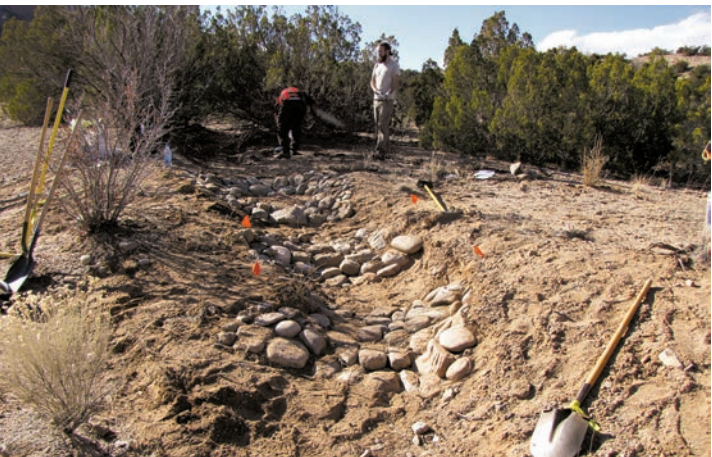
Examples of small rock structures (One-Rock Dams and Rock Bowls) during construction to stabilize a small gully.
