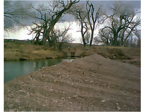
Repaired Diversion of Fort West Ditch. Photo by Linda Stailey.
