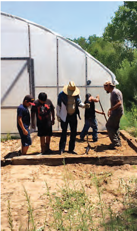
Youth and Mentors do a soil compaction dance to prepare the base for a large water tank. Photo by Juliet Garcia-Gonzales, NMAA Staff.
