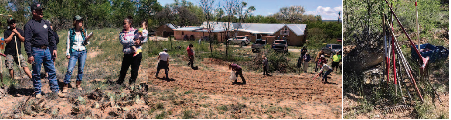
l to r: NMAA staff Serafina Lombardi and Donne Gonzales were part of the work crew removing elms and cactus. Entre mas manos, el trabajo es menos. Many hands, less work. In April, 25 people got together to restore a parcel of fallow land in Nambe. People brought their hand tools to restore land in Nambe, where there is intense pressure to keep water rights in beneficial use. Photo credit: NMAA
